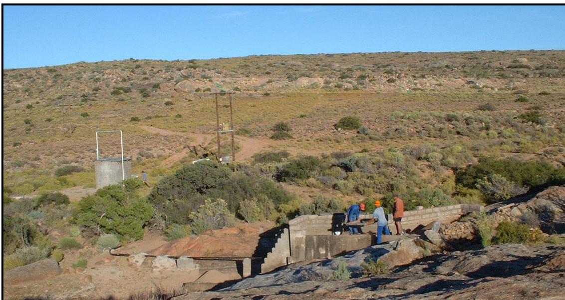
Figure B.16: Sand filter with injection and abstraction borehole (pump house) in the background
